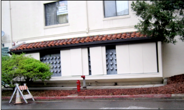
112 Smart Meters in apartment complex
