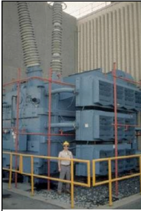
Generator step-up transformer damaged by March 1989 solar storm.
